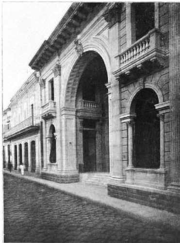
THE ROYAL BANK OF CANADA. At Havana, Cuba. The entire front of this building constructed of Stevens Cast Stone, while the foundations, side and rear walls are constructed of the Palmer Hollow Concrete building blocks.
