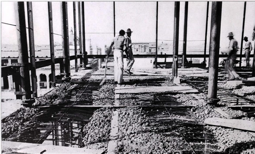
FLOOR ARCHING, HAVANA CIGAR FACTORY. Taken during Construction, showing Method of Constructing Floor Arches with Reinforcing Metal and Flooring in Concrete.
