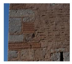
Figure 1. Benavites Tower (Valencia) 14-16th c. South corner detail with reused materials. Source: VLM
