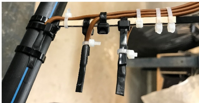
Fig. 5. Thermocouples with waterproof covers and a wiring system were fixed in position along with a wooden stick.
