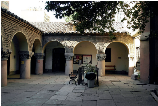
Fig. 18. General view of the main patio of the Casa de Los Diez. (Source: The author).
