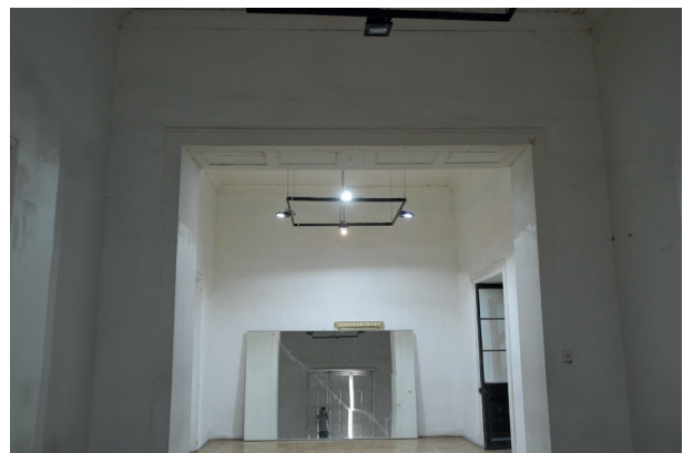
Fig. 12. Adobe walls in ground floor rooms. (Source: The author).
