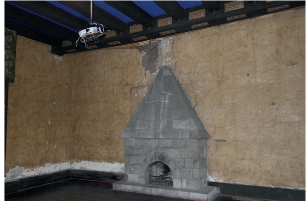
Fig. 11. Adobe walls in ground floor rooms. (Source: The author).
