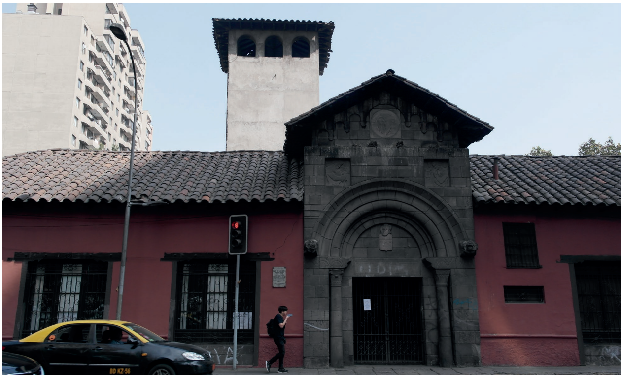
Fig. 3. Facade and main access of the "Casa de Los Diez", and inner tower, visit year 2019. (Source: The author).
