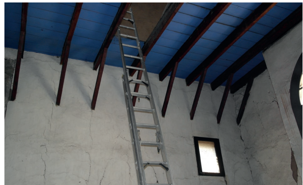
Fig. 17. Interior view tower walls, visit of the year 2019. (Source: the author).
