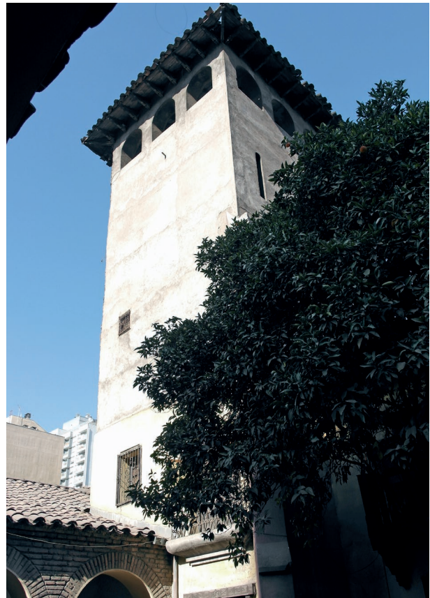
Fig. 16. Exterior views of the Tower, visit of the year 2019. (Source: the author).
