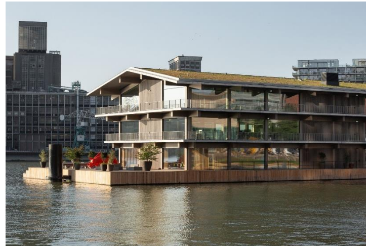
Figure 25 - The Floating Office, Rotterdam, Netherlands. Source [23]
