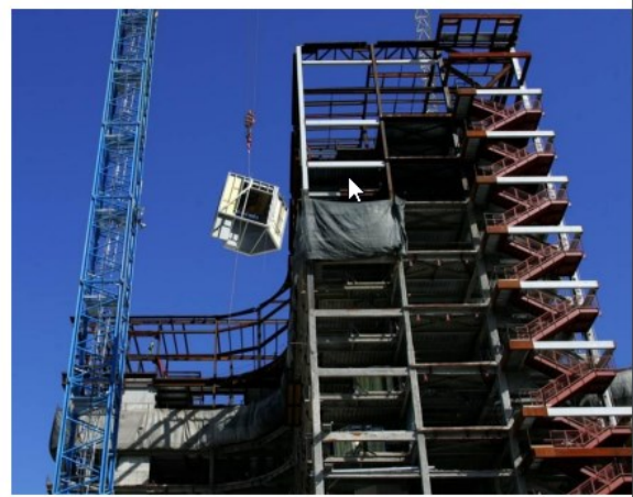
Prefabrication work complete: 12 October 2009
