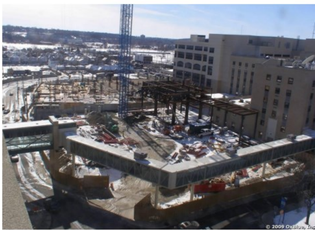
Prefabrication work begins: 2 February 2009
