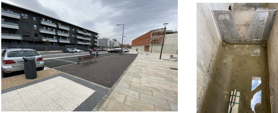
Figure 2. Image of the pavement site (left), with a parking area (darker asphalt) and walkway area (red pavers), and manholes for flow control (right).
