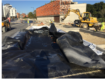
(b) Experimental site waterproofing.
