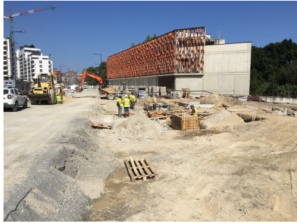
(a) Experimental site construction.
