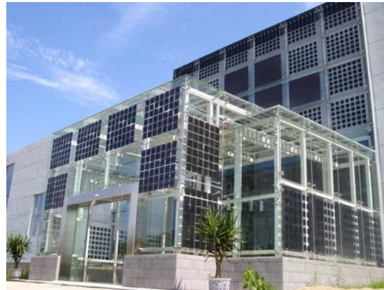
Figure 2.3: Transparent BIPV construction example [37].
