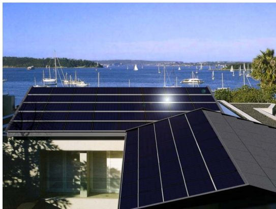
Figure 2.2: BIPV roof example [36].
