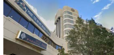
2 ASCENSOR ELDRORADO CASINO
