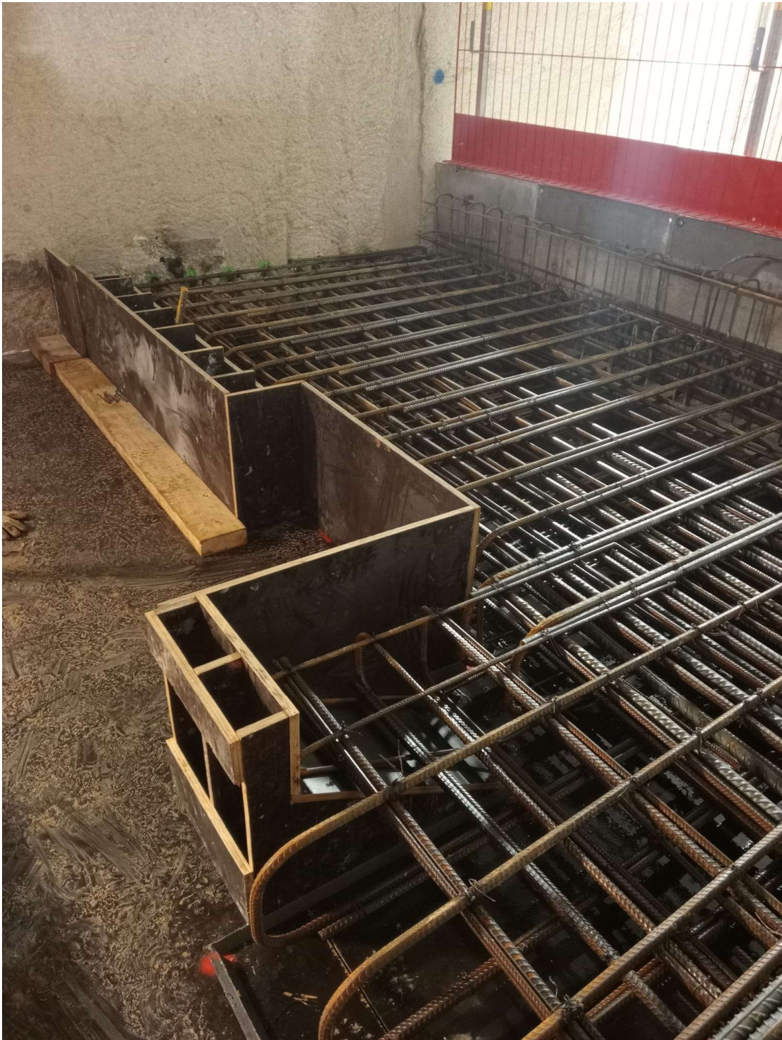
Figure 83. Coffrage biseau cage 10
