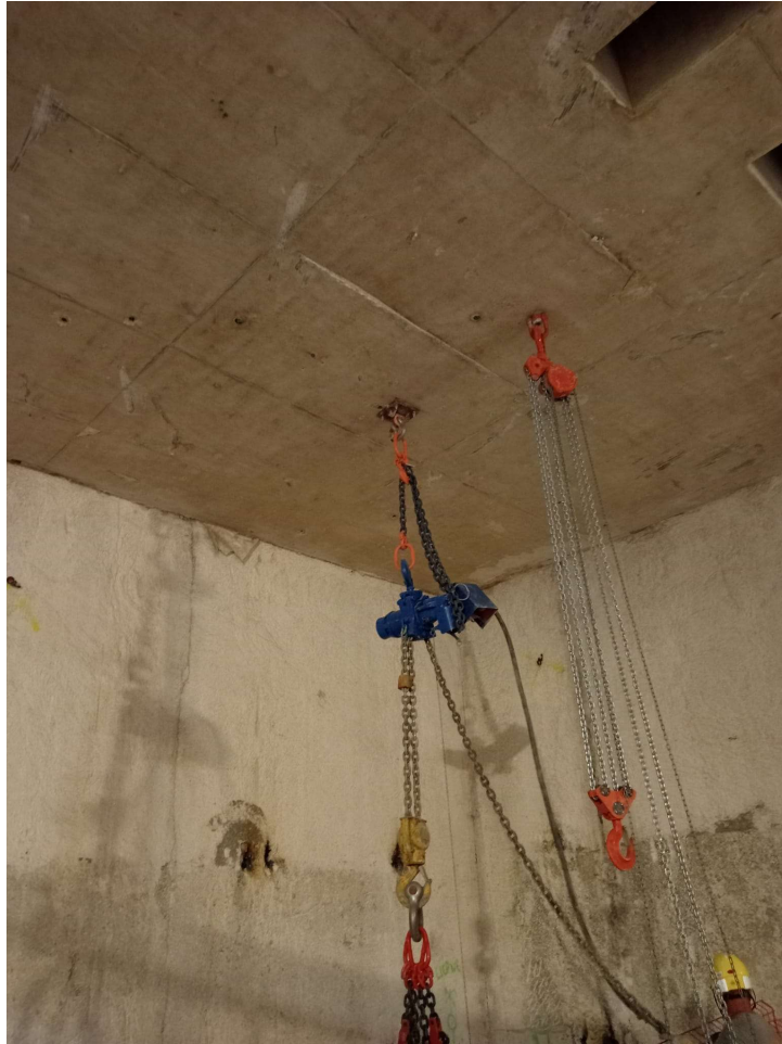
Figure 72. Plaque inserts 9B
