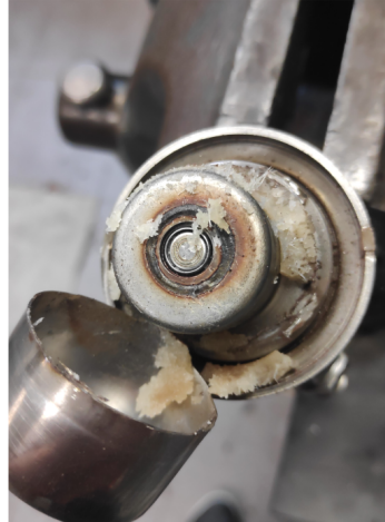
Figure 3.1: Urea deposits formed at the orifices of a UWS dosing module [10].
