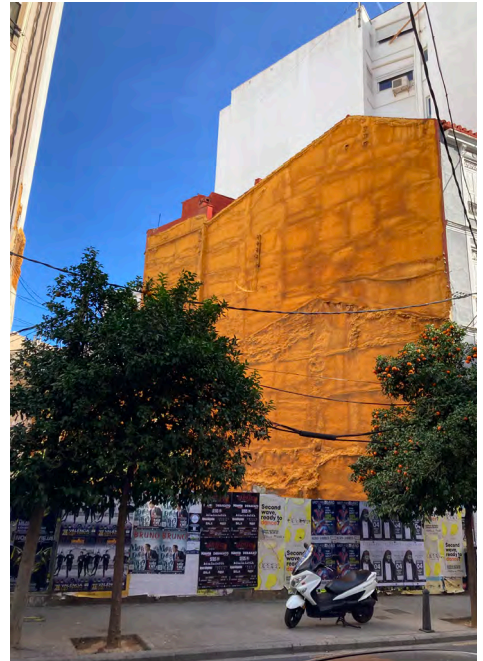
view of the building site
