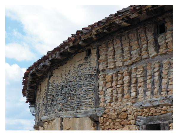
Figure 1. Example of a half-timbered wall with stacked masonry infill and wattle-and-daub screen, in La Cuenca (Soria). Source: Alicia Hueto Escobar.
