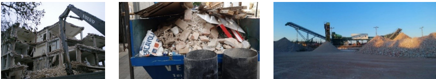
Figure 2. Non-selective demolition works, Pl. America, Valencia (2010), a container with different materials mixed and a recycling plant, where C&DW is sorted and classified. Source VLM
