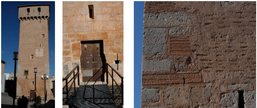
Figure 1. Benavites Tower (Valencia) 14-16th c. South corner detail with reused materials. Source: VLM
