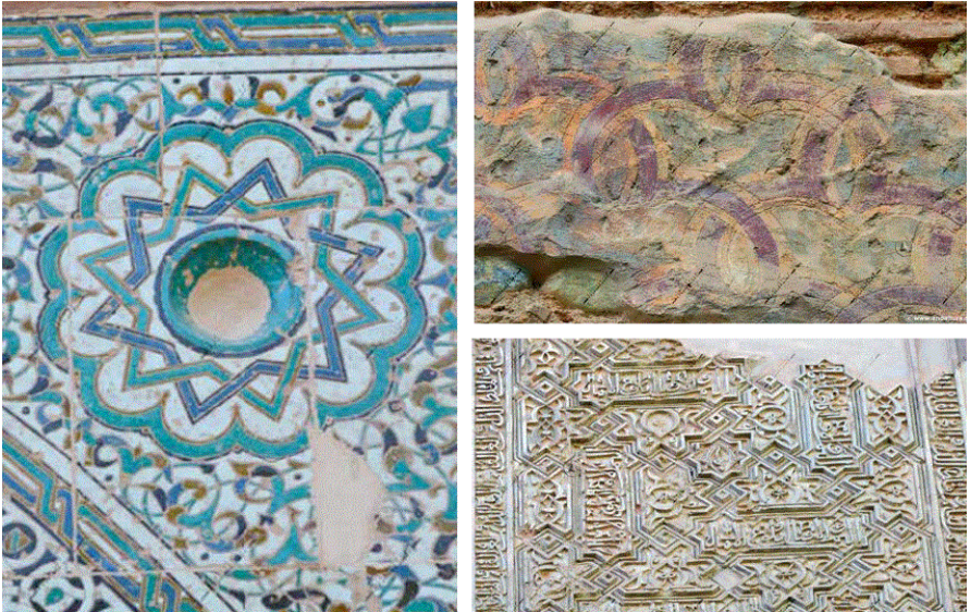
Figure 6. Detail of ornamentation on the Eastern facade of the Wine Gate (Alhambra, Granada): arabesque in spandrels ( albanegas ), plasterwork and remains of paint on plaster (Source: https://andaltura.com/la-alhambra-y-el-generalife/puertas-de-la-alhambra-y-el-generalife/puerta-del-vino/ ).
