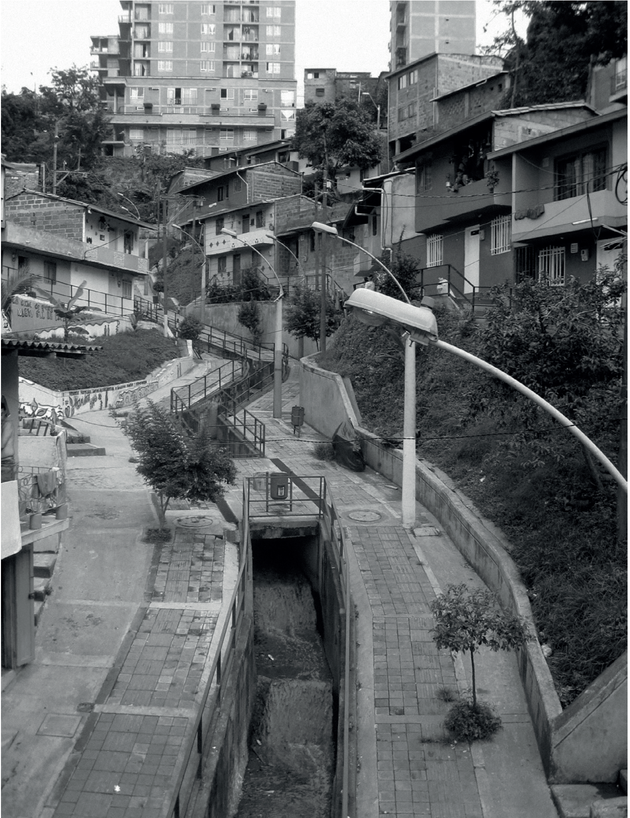
Figure 4 | Urban improvements and relocation housing in Quebrada Juan Bobo, Comuna Nor-Oriental, Medellín, Colombia. Photo: David Gouverneur.
