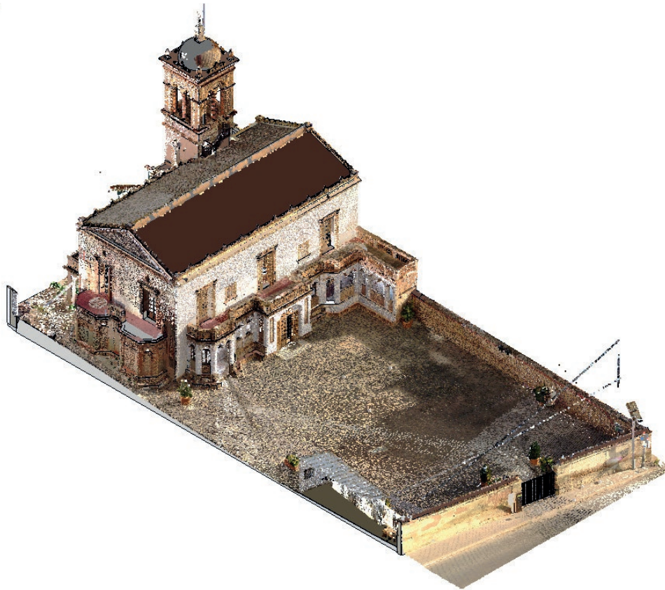
Fig. 9. Overlap of the point cloud with the model in Revit (Source: Esteve Muñoz).
