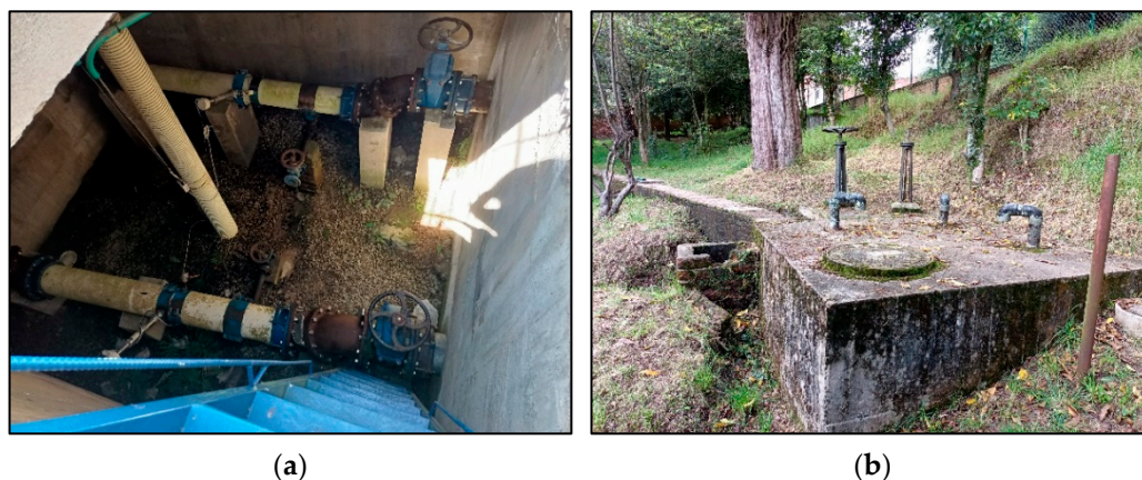
Figure 5. Record of field inspections. (a) Piping and valves; (b) pressure-bursting chamber 4.
