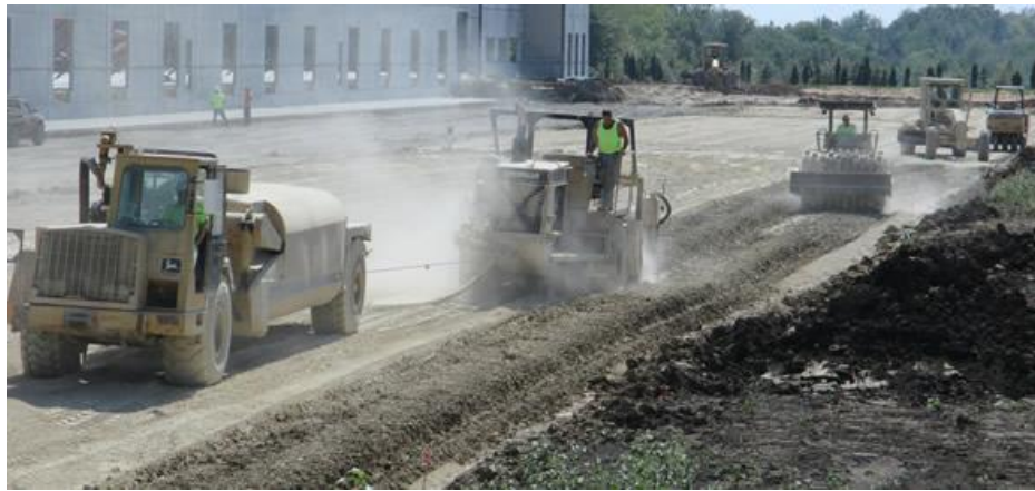
Figure 60. Stabilization with fly ash procedure. Source: Fly ash stabilization steps (KCFA,2012)
