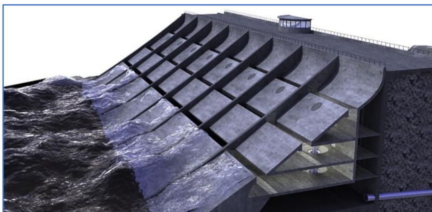
Figure 1. Sea slot-cone generator (SSG) [17].
