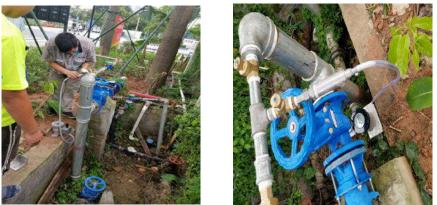
Figure 5. Pressure gauge installation at critical node
