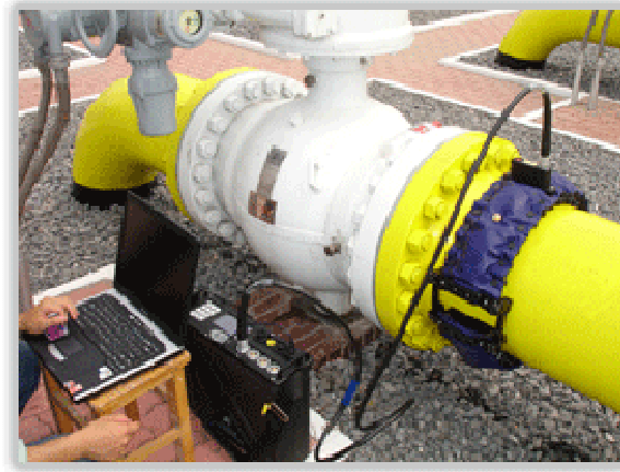
Figure 8. Guided Ultrasonics, Ltd. probe attached to a pipe (source: GUL Ltd, 2011)
