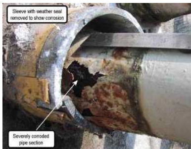
Figure 11. Sleeved road crossing
