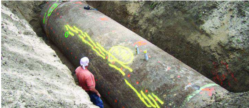
Figure 36. Buried pipe inspection by visual method with magnification (source: Rosen Ltd , 2011)
