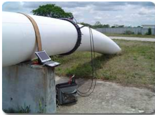
Figure 24. Guided Waves buried pipe examination (source: GUL ldt , 2011)
