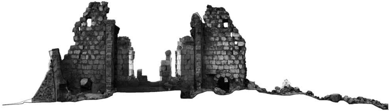
Figure 8: A photomontage of the current state of the main front walls of the Western Basilica.
