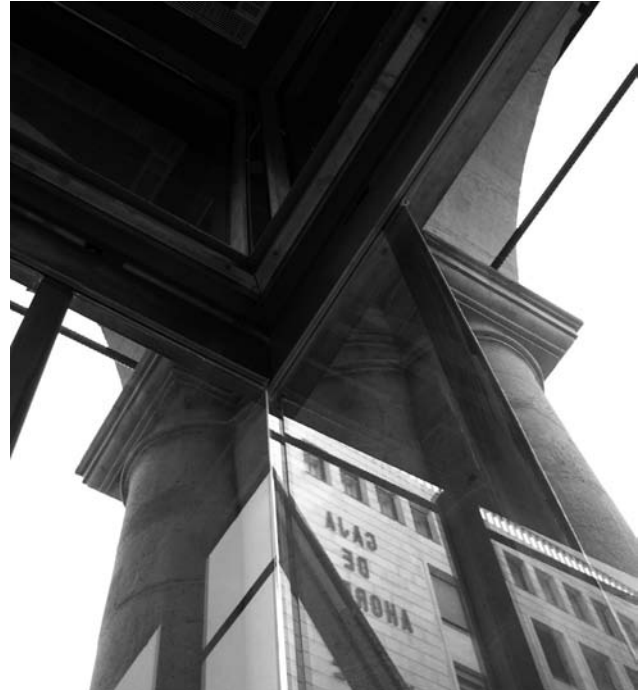
Figure 18: Interior view of the corner intersection
