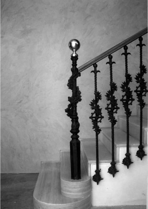
Figure 5: Curtail on the stairs
