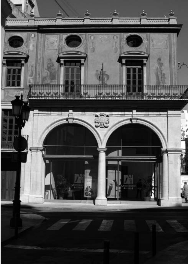
Figure 7. Image of the facade from Colón street
