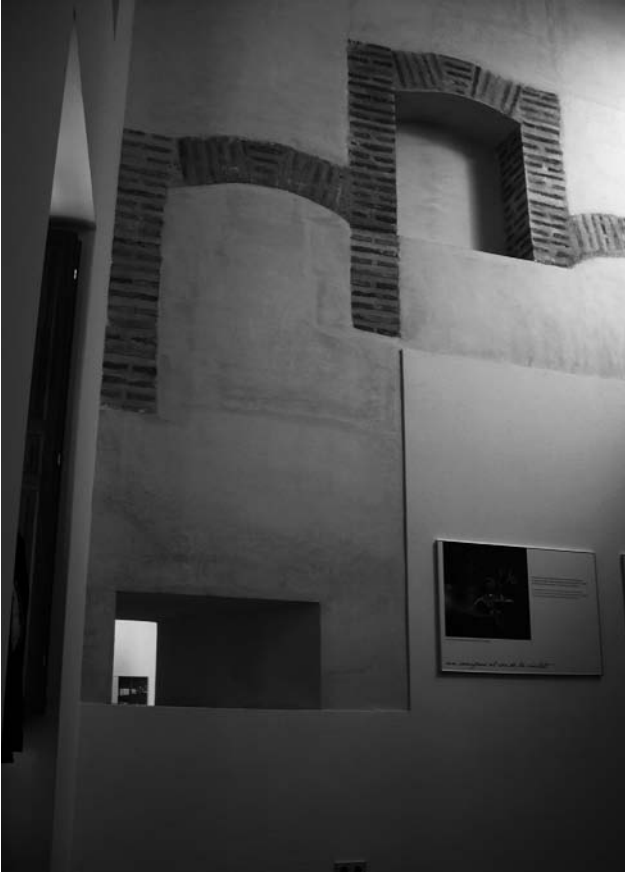
Figure 11: Remains of the old facade on an interior wall of the Llotja
