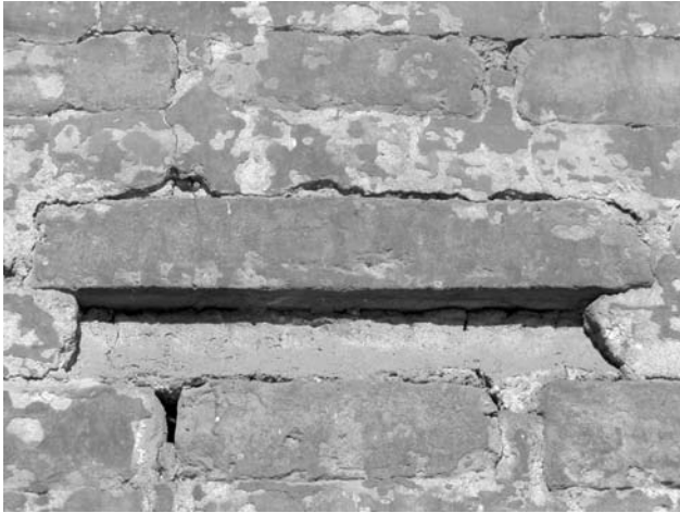
Figure 3. San Andrés church. Detail of the double joints in the masonry of the front of Calle Procida. First part of 17th century
