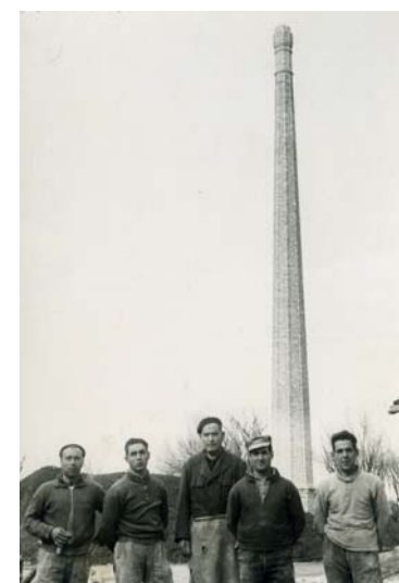
Figura 6.164: Chimenea alcoholera Domecq, Villacañas (Toledo)
