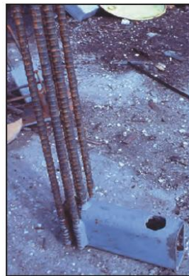
(c) Steel tube bearing support viewed from the top
