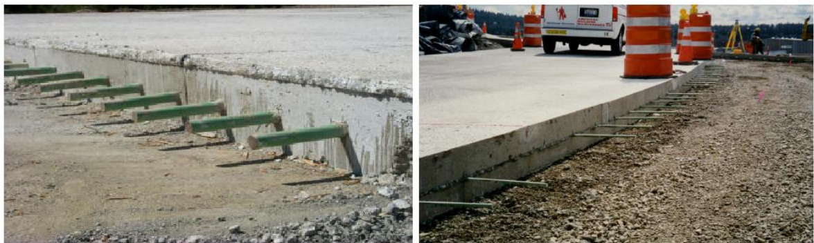
Picture 33 - Dowel bars in the left picture and tie bars in the right
