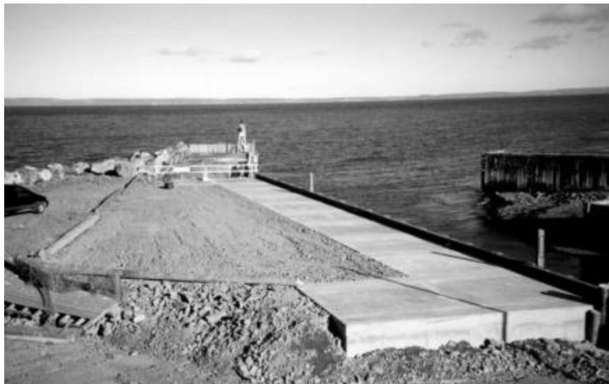
Figure 7 [25], Picture of Hall's Harbor after rehabilitation
