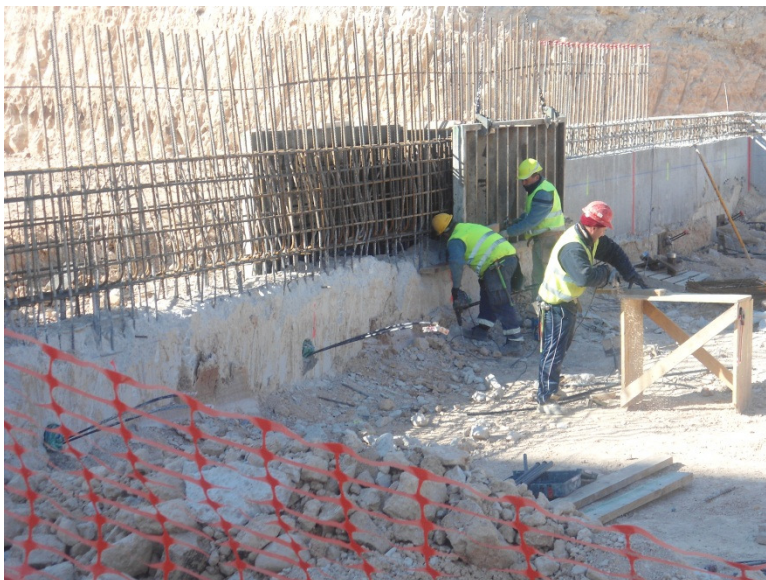
(P71: Demolition and replacement of the top layer)
