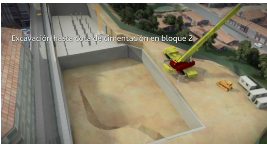
(P88: Excavation till foundation floor in block 2)
