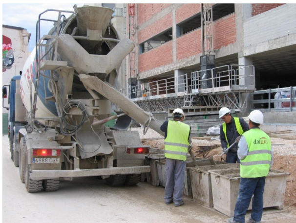
(P9: Delivery of concrete)
