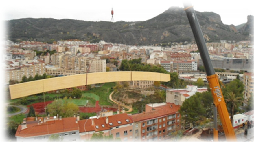
(P57: Telescopic crane used to lift the wood beams)
