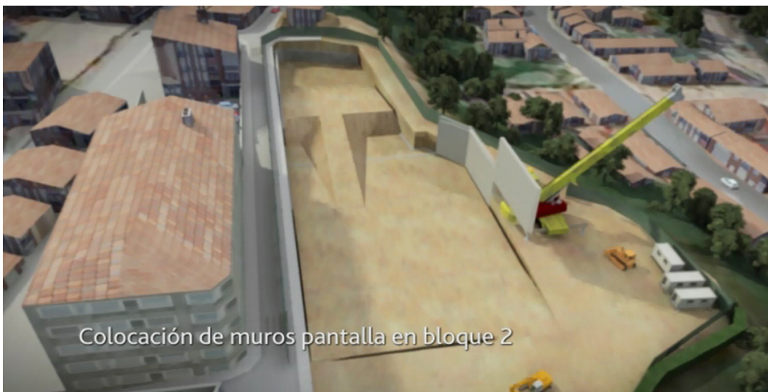
(P84: Construction of diaphragm walls in block 2)
