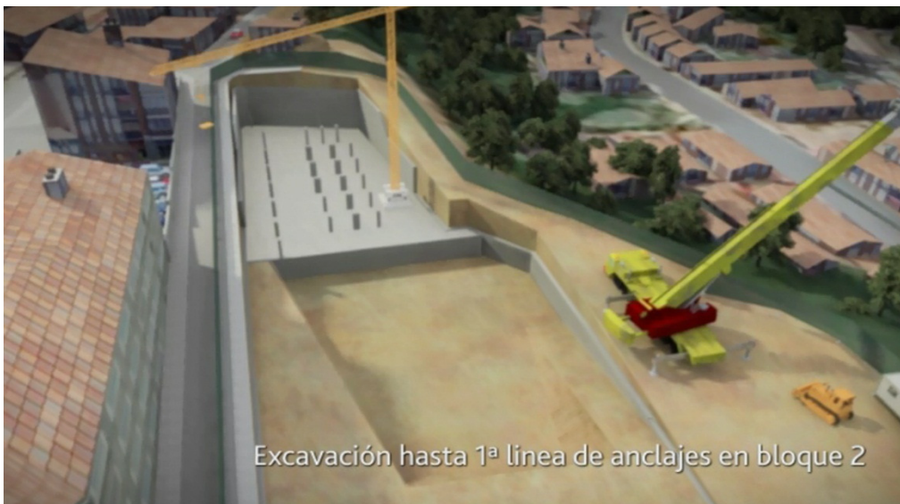
(P87: Excavation part 4 till anchors in block 2)
