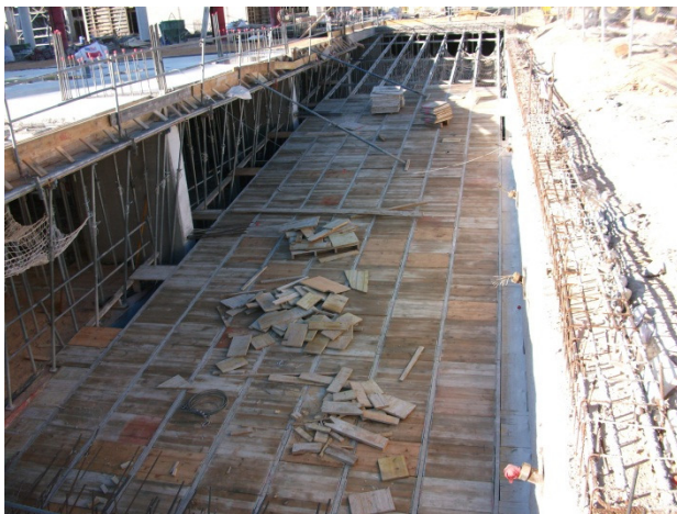
(P53: Wood molds, ramp)
