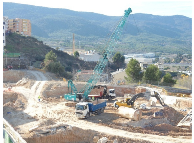
(P16: Excavation of the ground)
