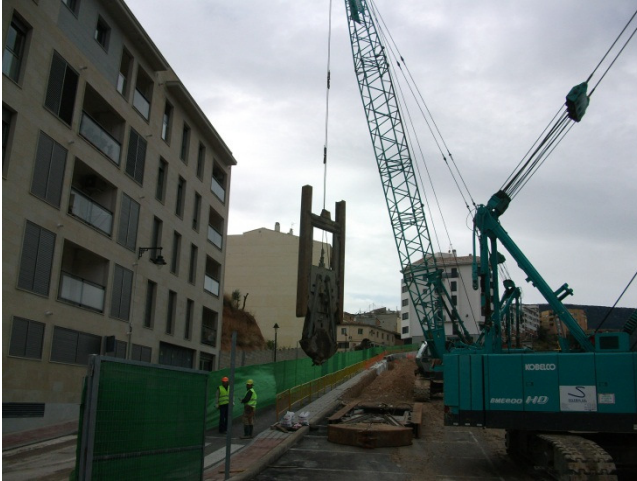
(P27: Diaphragm wall excavator)
