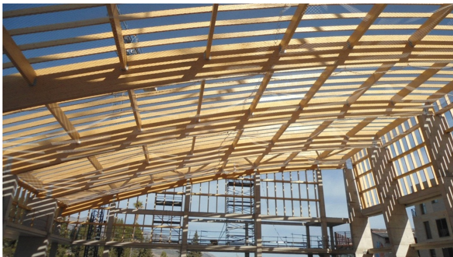
(P58: Wood structure, sports hall)
