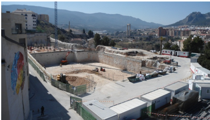
(P22: Diaphragm walls)
