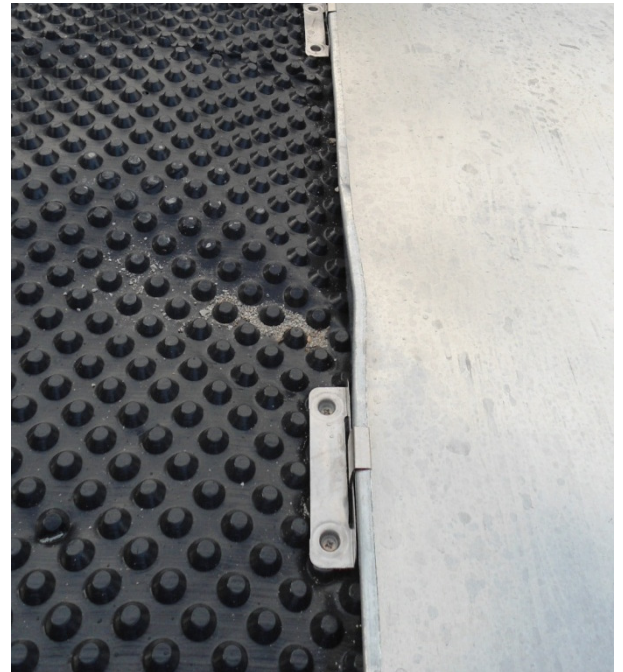
(P60: Detail draining sheet, naps)
