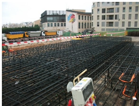
(P70: Steel reinforcement cages)
