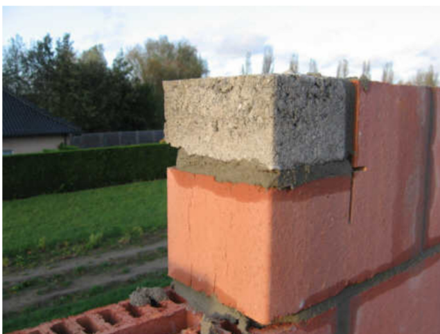
(P96: Carpentry Belgium)
