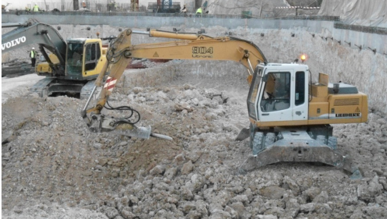
(P20: Backhoe with jack hammer)
