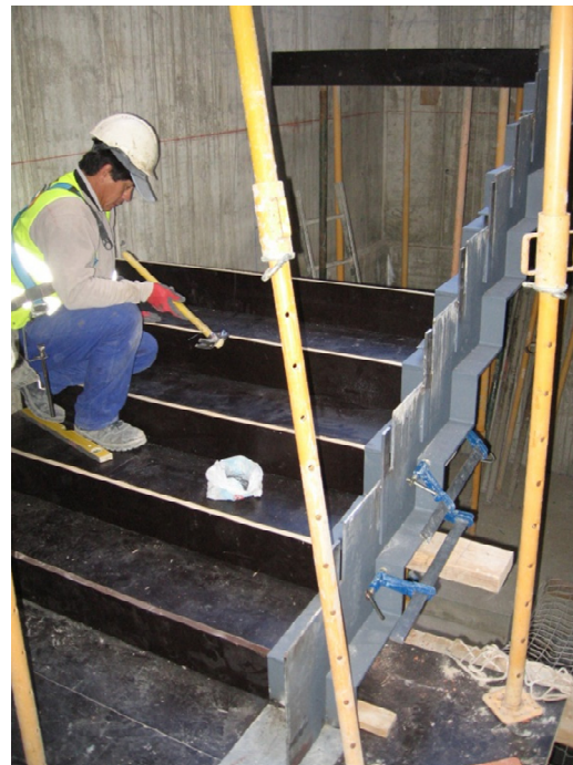
(P56: Central staircase wood formwork)
