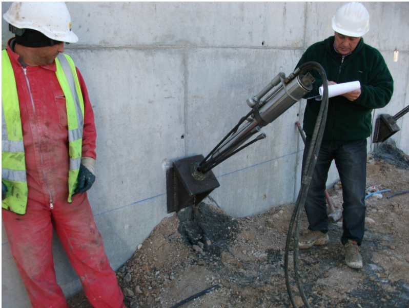
(P76: Tension anchors)
