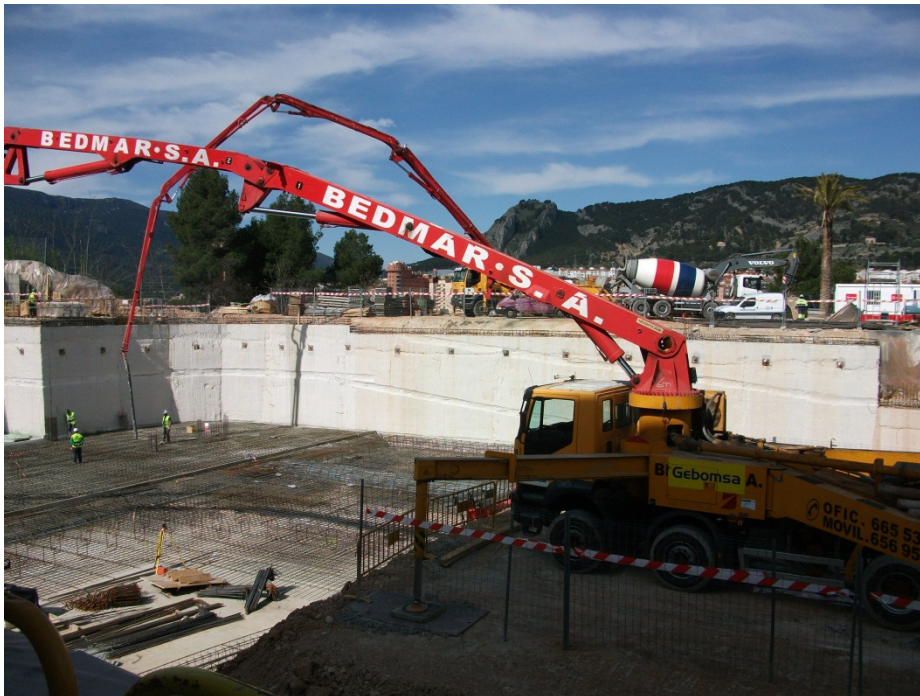
(P29: Concrete pump in action)
