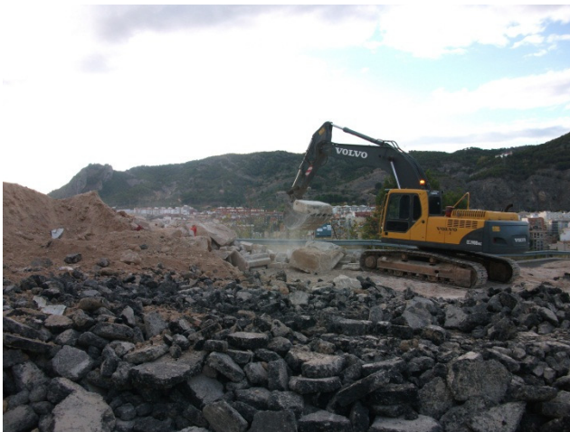
(P15: Removal of the asphalt and pavements)
