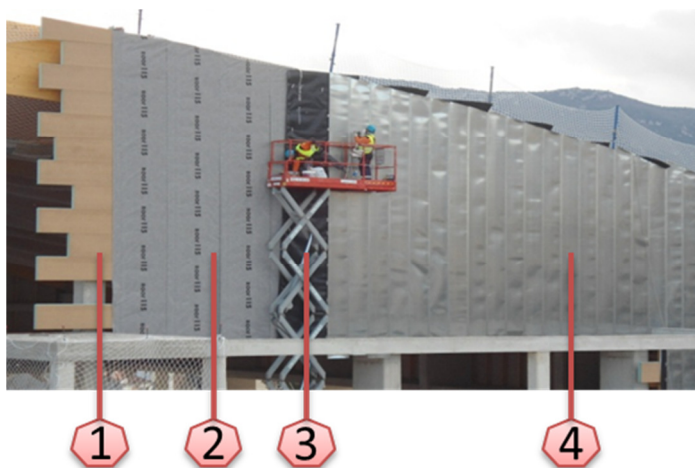
(P59: Exterior roof side coverage, sports hall)
