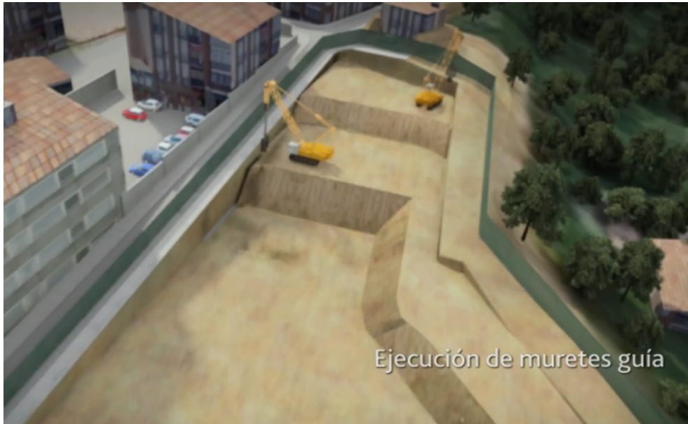
(P81: Construction guide walls)
