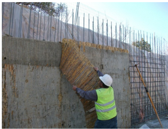
(P48: Reed structure molds)
