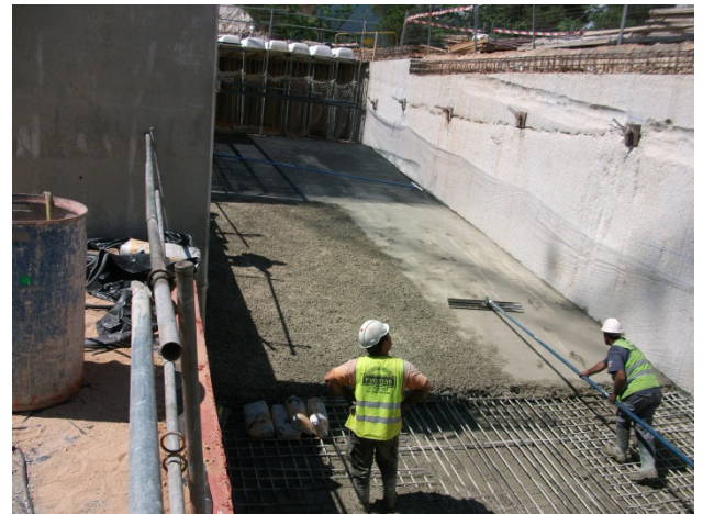
(P54: Nerves into the surface for more grip)
