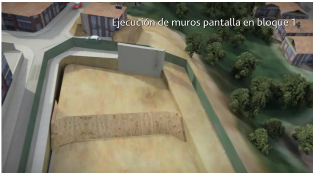
(P82: Construction of diaphragm wall block 1)
