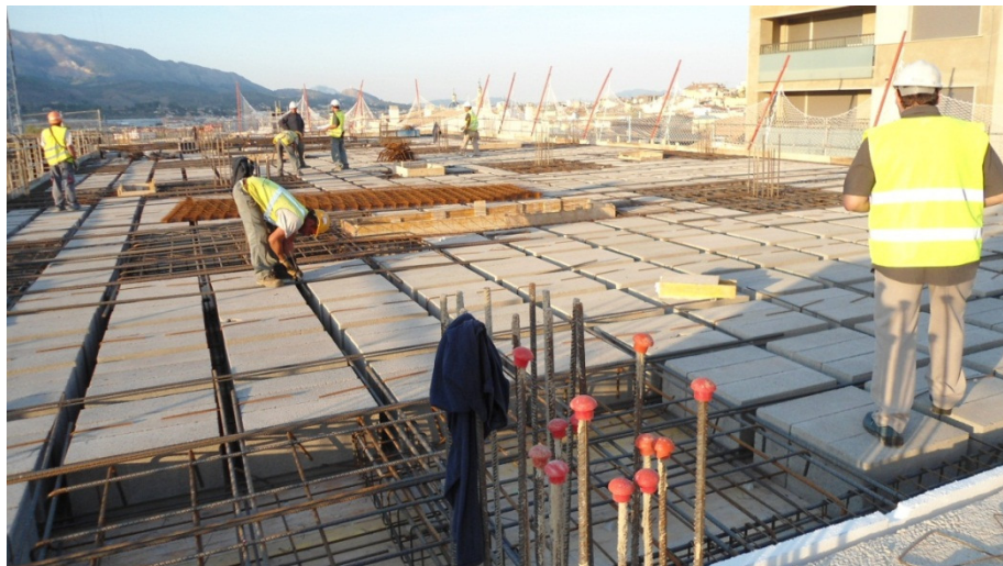
(P47: Concrete blocks set in place)
