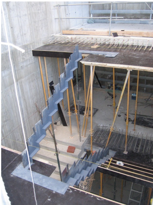
(P55: Central staircase steel mold)
