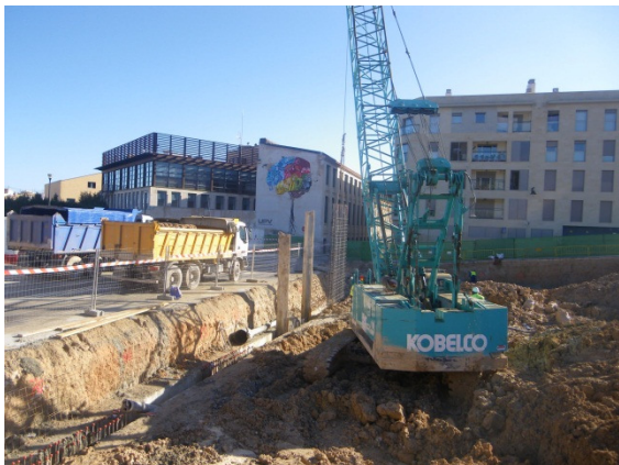
(P63: Kobelco slurry wall excavator)
