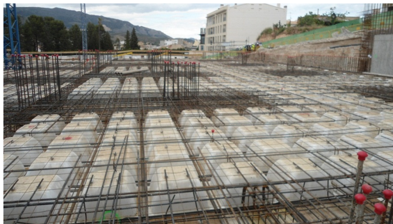
(P45: Plastic coffers set in place)
