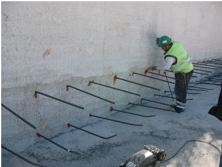
(P78: Glued reinforcement)
