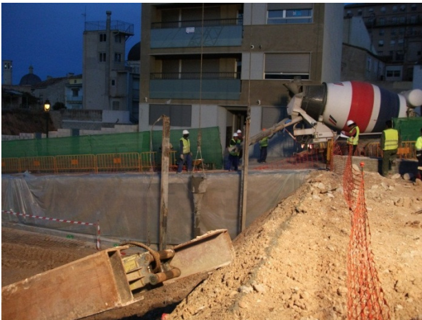
(P25: Diaphragm walls being filled with concrete)
