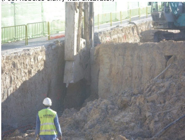
(P64: Slurry wall excavator claws)
