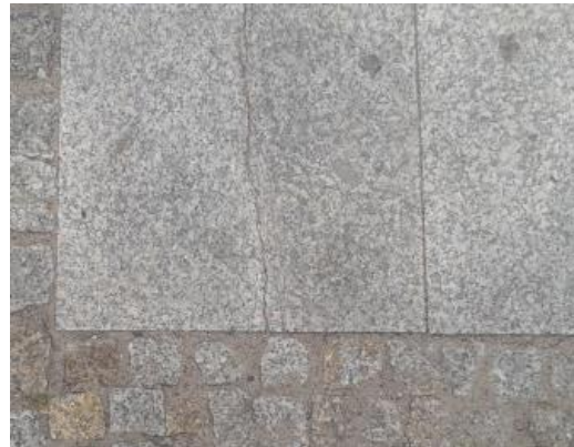
Fissures by climatic causes: Valencia (picture 1), Szczecin (picture 2) [1]
