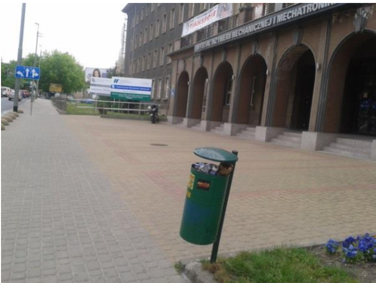
Pavement renewed in access to the faculty of Mechanical Engineering [3]
