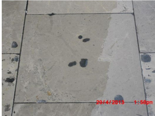
Presence of surface deposits over the pavement:Valencia (picture 1), Szczecin (picture 2) [1]
