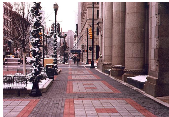
Helsinki Street without snow with under floor heating [2]
