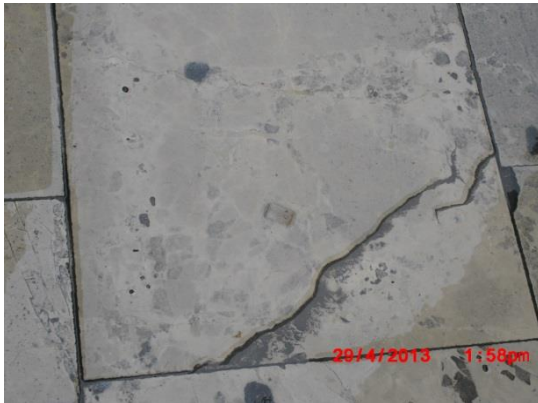
Fissures by climatic causes: Valencia (picture 1), Szczecin (picture 2) [1]
