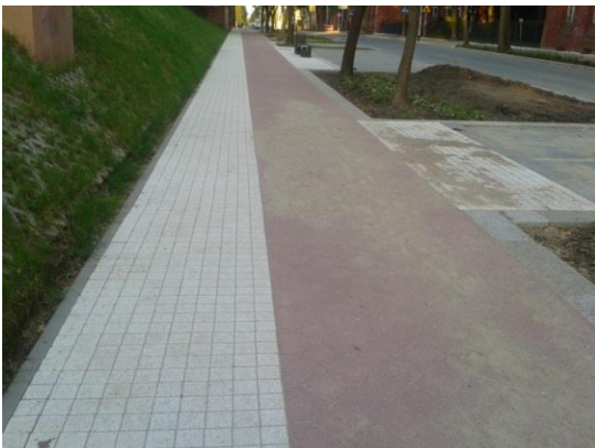
Renovated sidewalk Sowinskiego Street [3]
