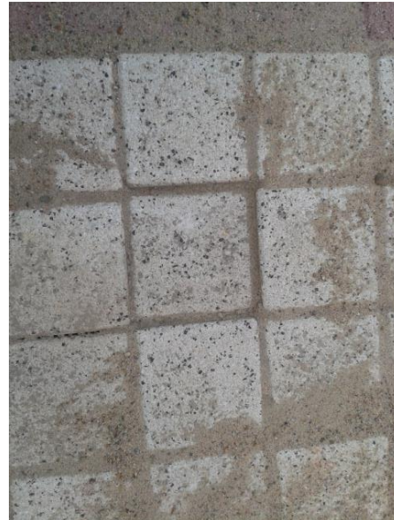
Joint execution difference: Valencia (picture 1) with mortar joints, Szczecin (picture 2) with sand joints. [1]
