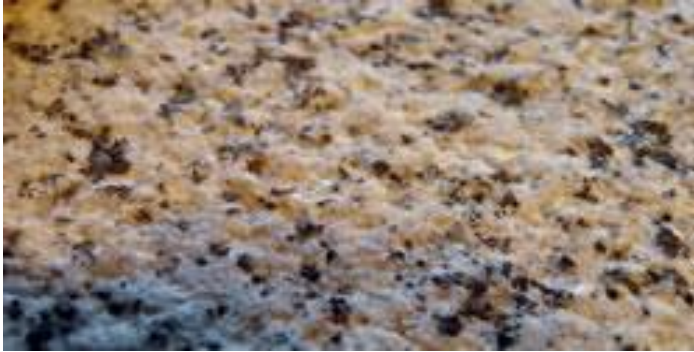
Bush hammered finish granite surface [5]
