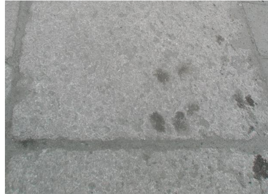
Presence of surface deposits over the pavement:Valencia (picture 1), Szczecin (picture 2) [1]
