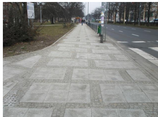
Replaced pavement in Szczecin' sidewalks. [3]
