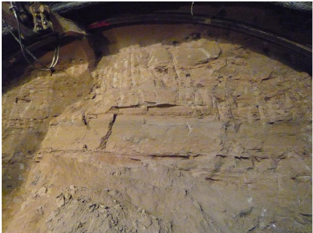
53 Fig. 4. Excavation front in progress, presenting high homogeneity and good stability
