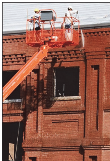
Figure 52. Example of water washing
