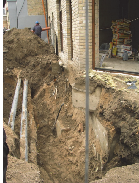
Figure 64. State of the courtyard walls and foundation during the waterproofing works
