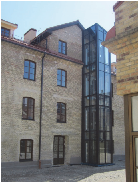
Figure 8 . Picture of the courtyard elevator after reconstruction works
