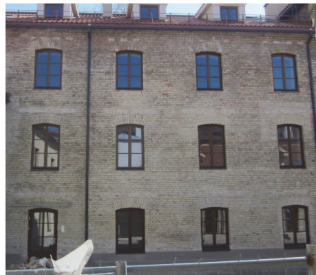
Figure 71. Courtyard facade of eastern wing after the reconstruction works
