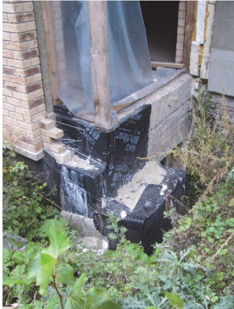
Figure 63. State of the courtyard walls and foundation during the waterproofing works
