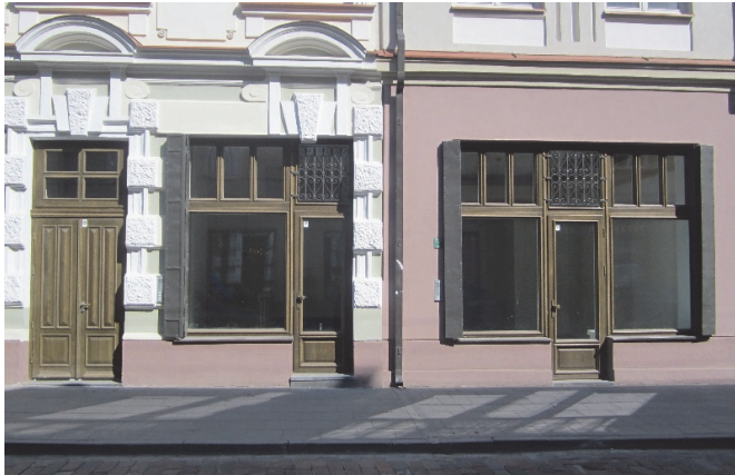
Figure 77. Protection grille installed in Traku Street facade
