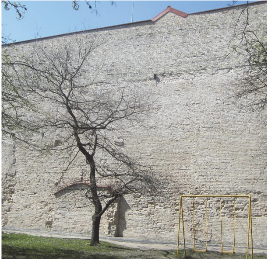
Figure 62. Exterior eastern wing facade after the reconstruction works
