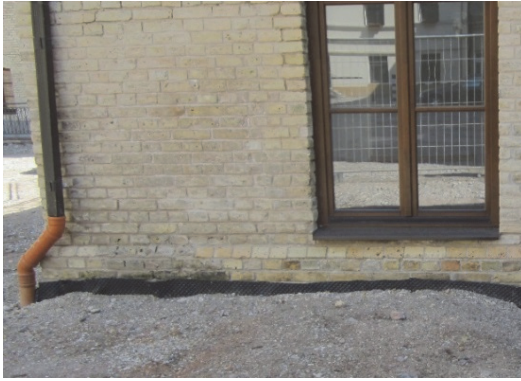
Figure 66. Foundation waterproofing installed after the reconstruction works
