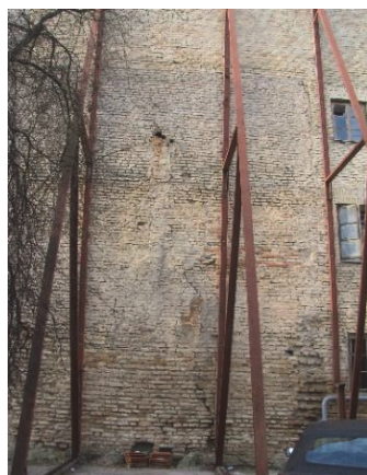
Figure 58. Exterior eastern wing facade before the reconstruction works
