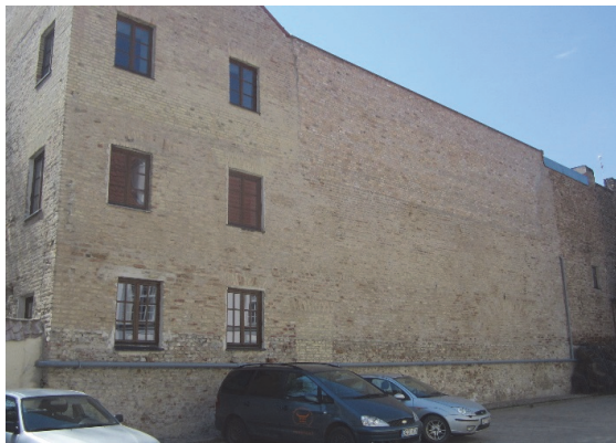
Figure 70. Exterior facade wall of northern, eastern wing after the reconstruction works
