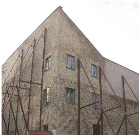
Figure 72. Exterior facade wall of northern, eastern wing, after first reconstruction
