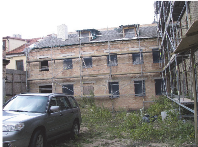
Figure 73. Courtyard facade of northern wing, after first reconstruction
