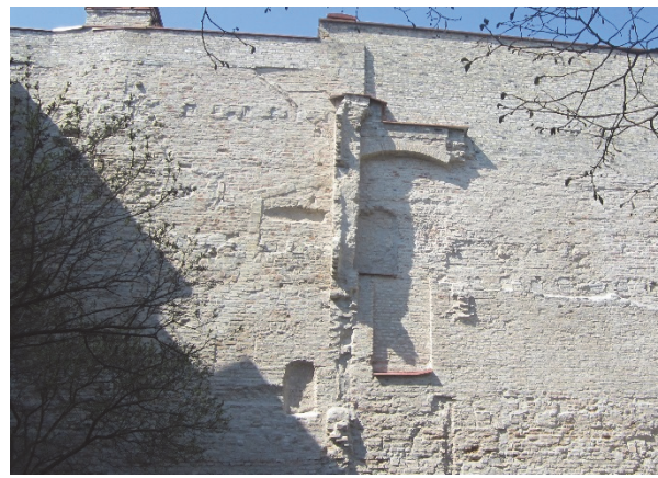
Figure 54. Exterior wall facade, picture after the restoration
