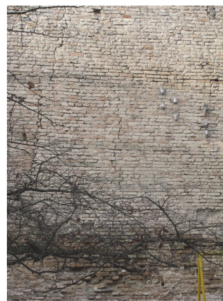
Figure 57. Exterior eastern wing facade before the reconstruction works
