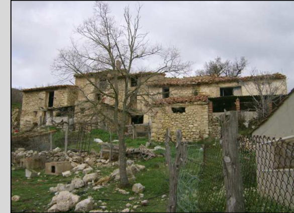
Fig. 6 Vista fachada principal
