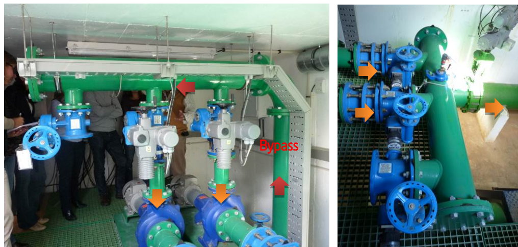
Figure 10.3: View of the pump as turbine installation
