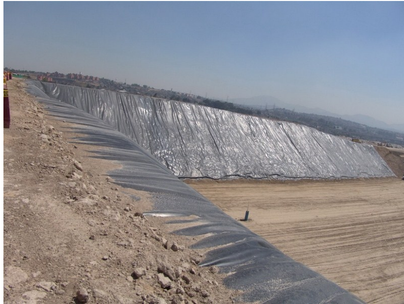
Figure 5.14 Tailings pond construction.
