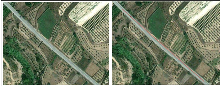
Figure 130. Low-deflection angle curve. The heading methodology allows us to detect this kind of curves.
