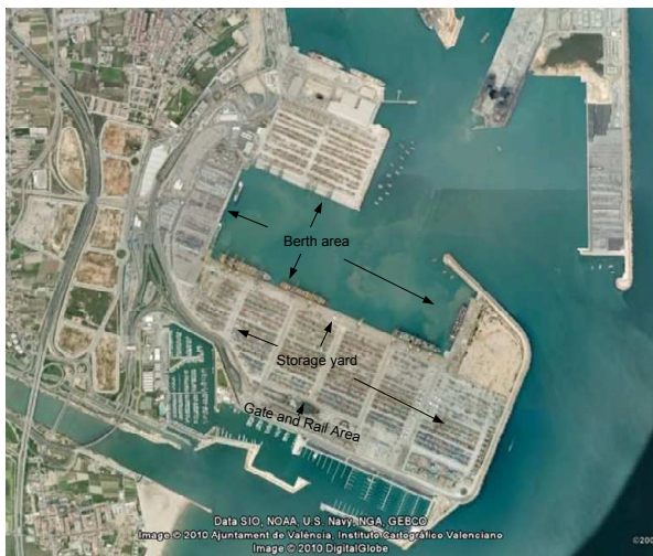
Figure 1: Container Terminal at Valencia
