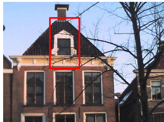
Image 10.2.5-2 Window of the attic
