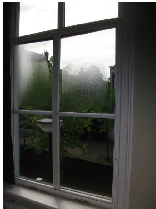
Image 10.2.4-6 Condensation on the window.
