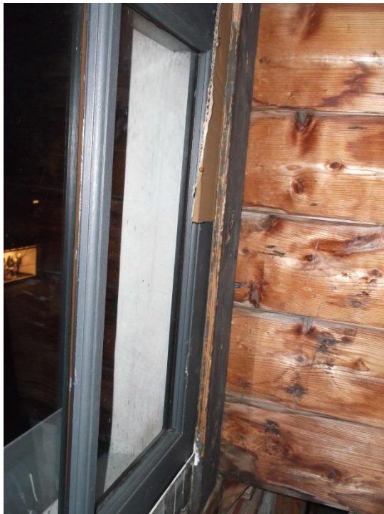
Image 10.2.5-1 Papers in the joints of the window
