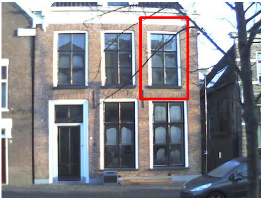
Image 10.2.4-4 Condensation on all the window
