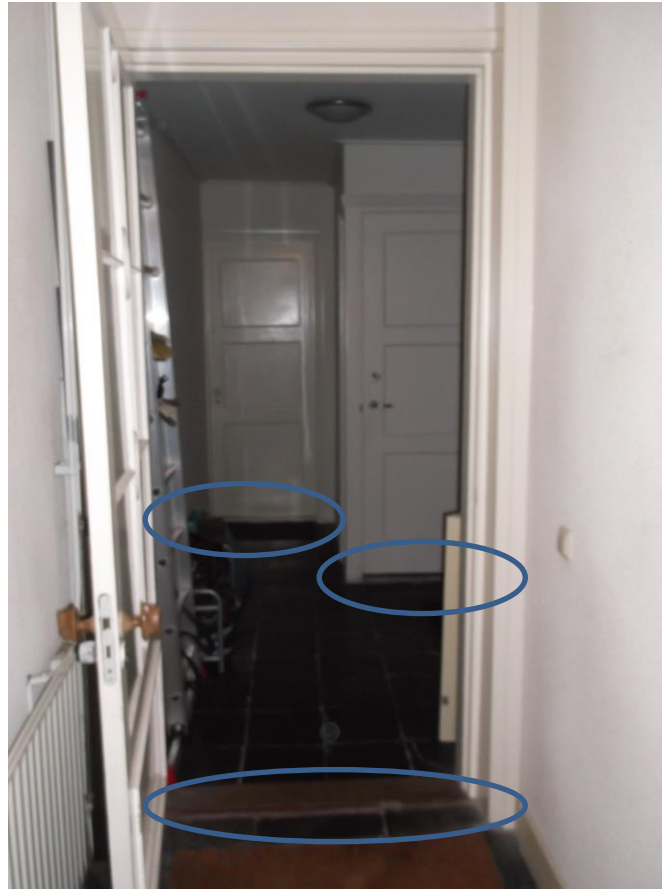
Imagen 14.1.2-2 Small stair between the level of the door and the tiling concrete.
