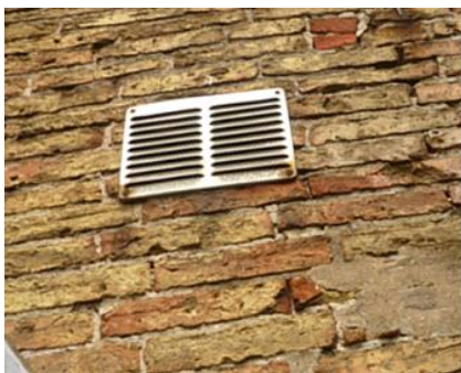
Image 12.2-1 Metal grill of the dryer (left facade)
