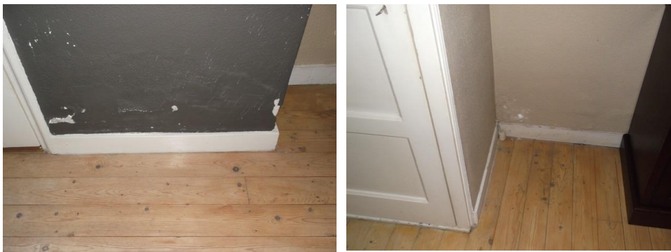
Image 9.2.1 Humidity capillary at the living room
