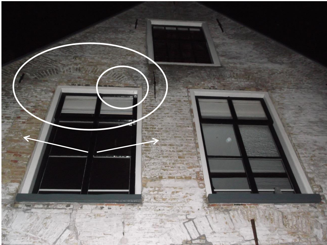
Picture 4.7.1.- North façade of the building
