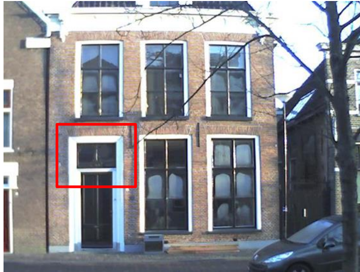
Image 10.5.2-3 Window A. Without condensations at the coldest part of the year
