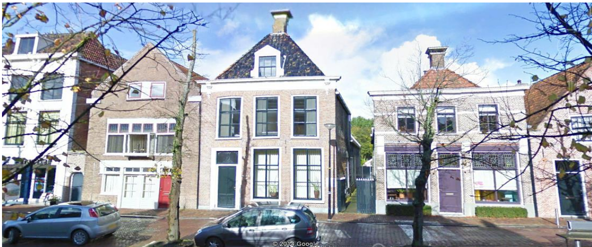
Image 3.2.3- Building of the project (At the middle)
