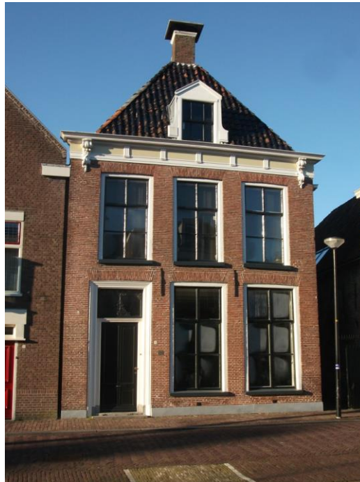
Image 4.3.1- Main facade of the building
