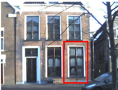
Image 10.2.2-5- Window C full of condensations
