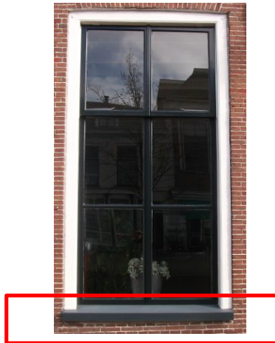
Image 10.5.2-1 Stone sill at the lowest part of the window
