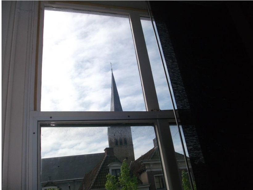
Image 10.2.3-1 Extra glass layer, on the low part of the window
