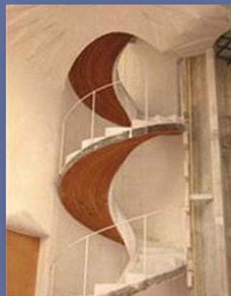
Figure 48. Staircase: example of Helicoid in Sagrada Familia
