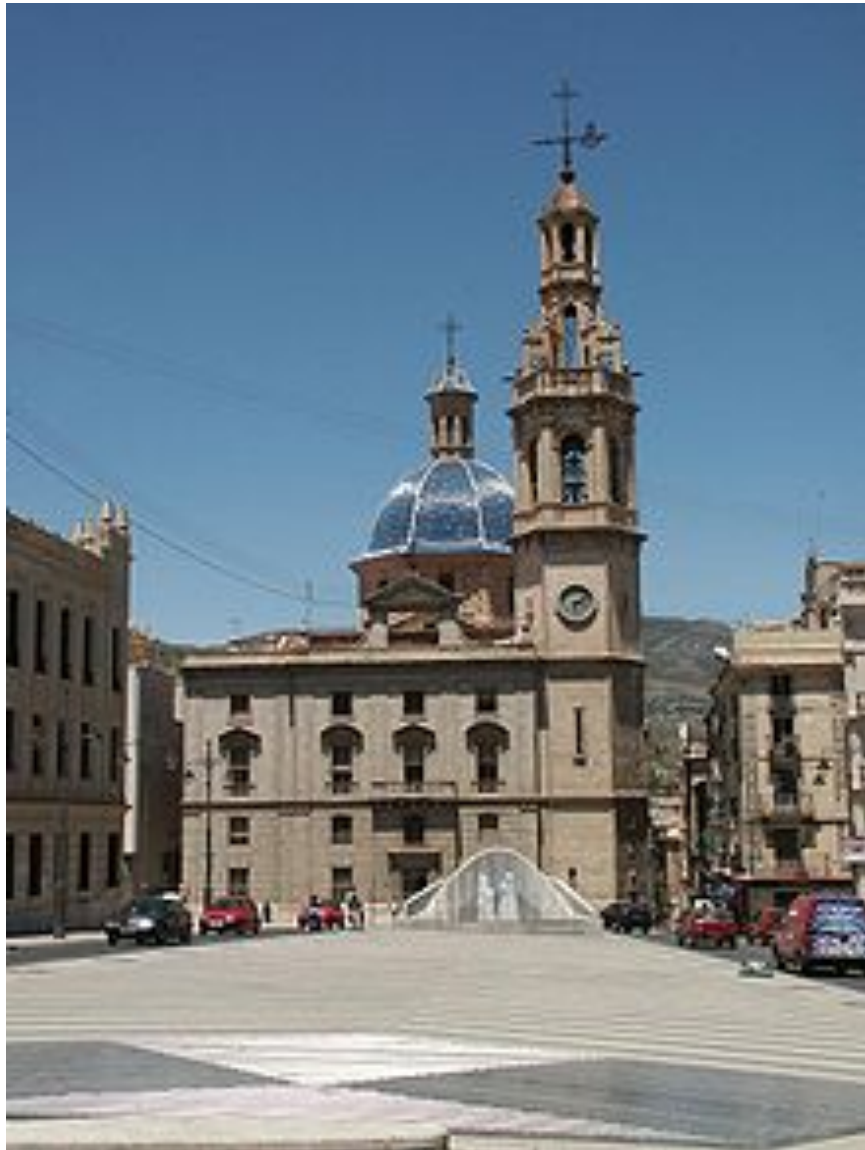
Pic. 3.1.4.6 Blue smelted tiles over dome
