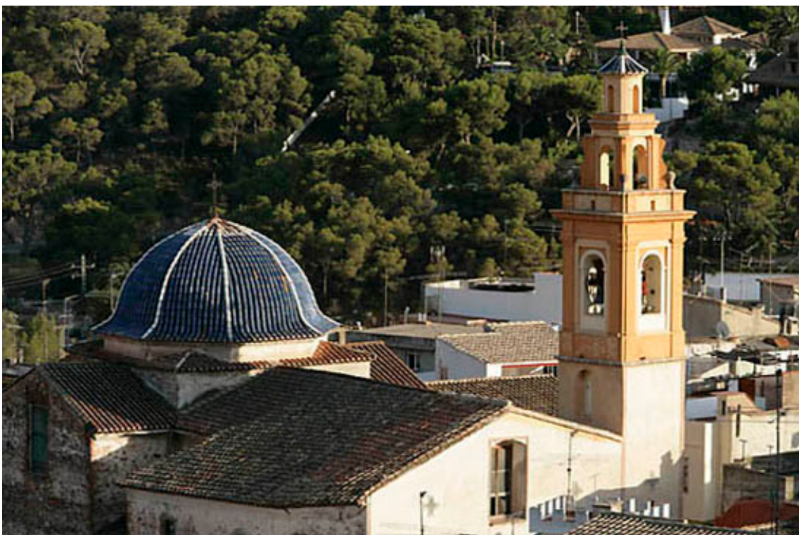
Pic. 3.1.4.6 Blue smelted tiles over dome (Serra, Valencia, Spain)
