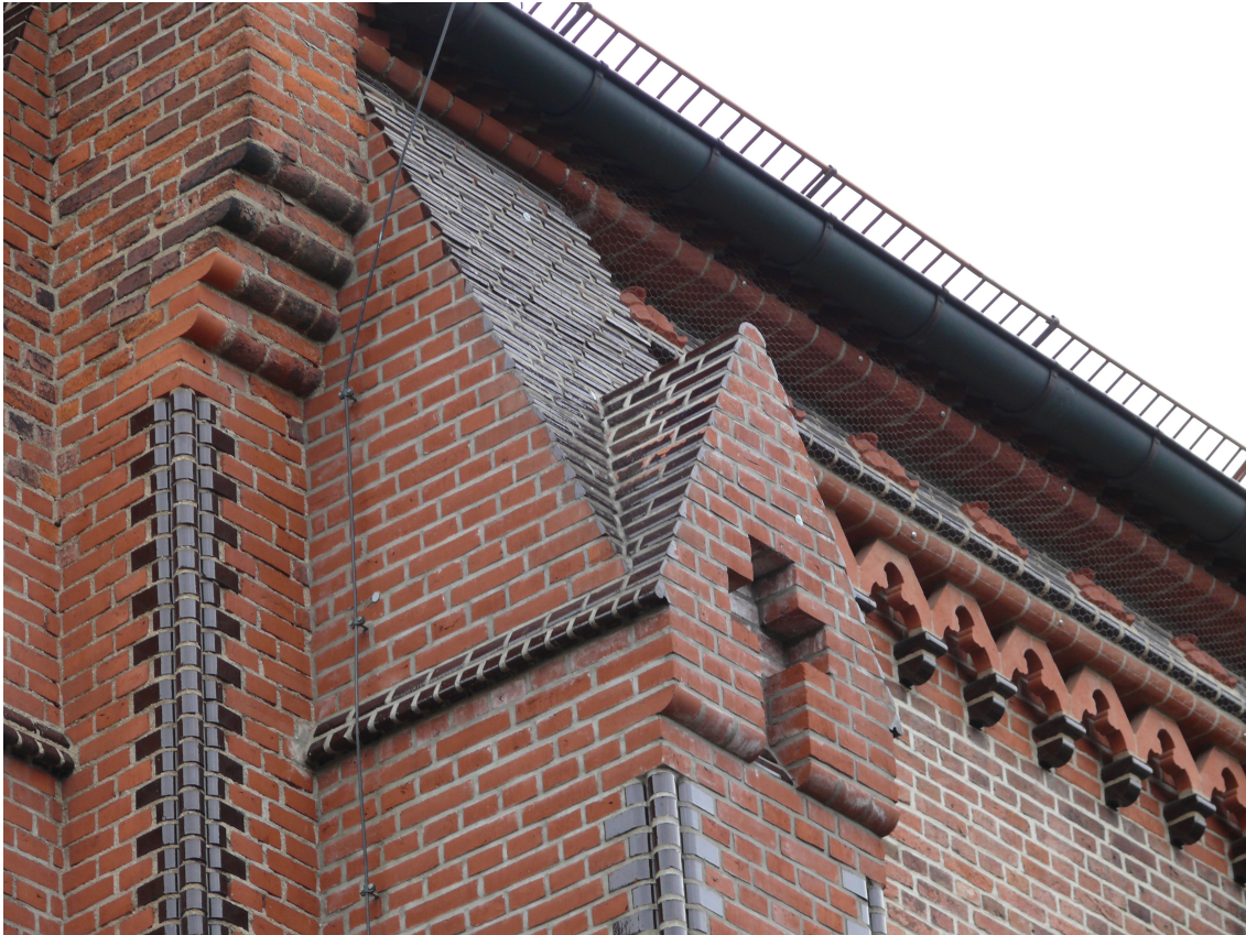
Pic. 3.2.1.2. Top of the buttress.
