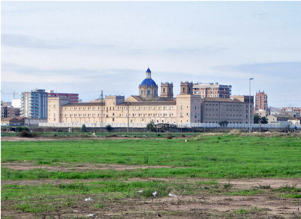
Pic. 3.1.4.7 Blue smelted tiles over dome
