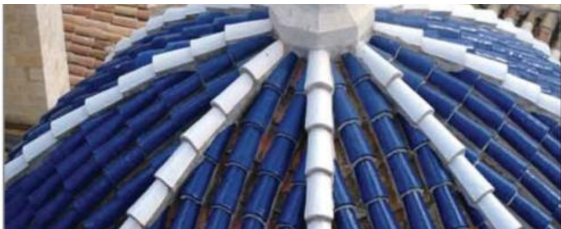
Pic. 3.1.4.5 Blue smelted tiles over dome.
