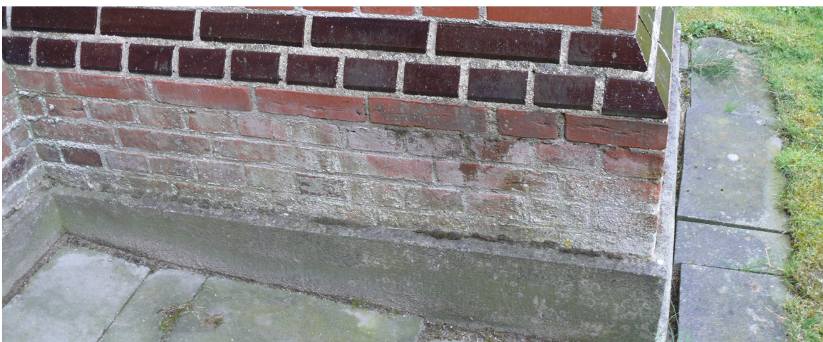
Pic. 3.2.1.6. Humidity from the ground
