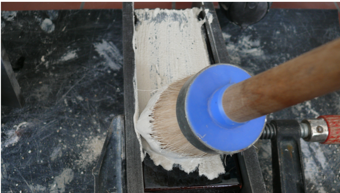
Pic. 3.3.1.11 Painting the surface with glue mortar.
