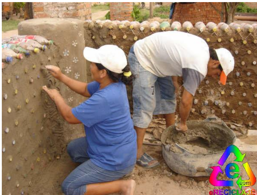
Picture. People building up a house with Ecobricks
