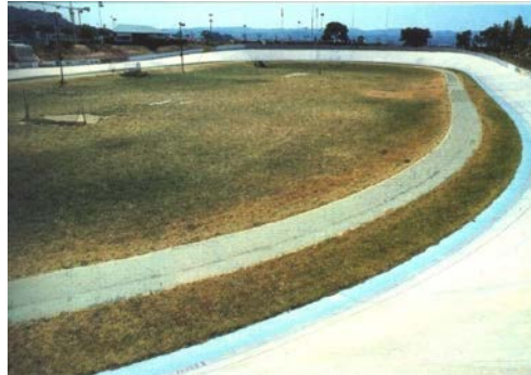
a) Infiltration basin
