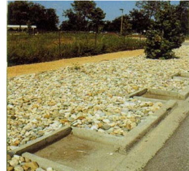
b) Infiltration trench
