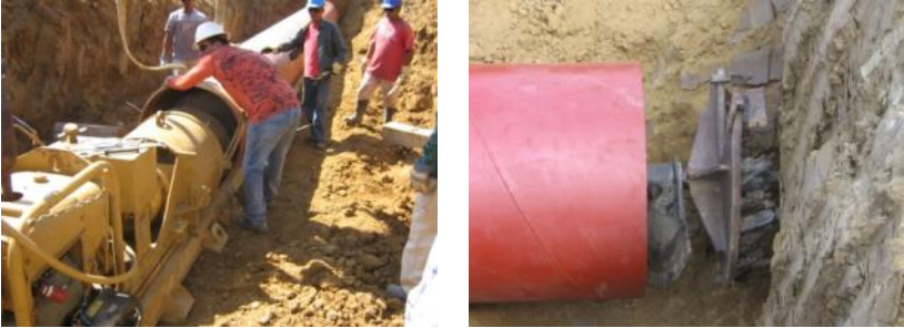
Soil boring and new pipe installation
