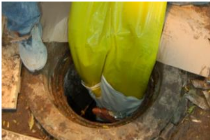
Initiation of lining installation
