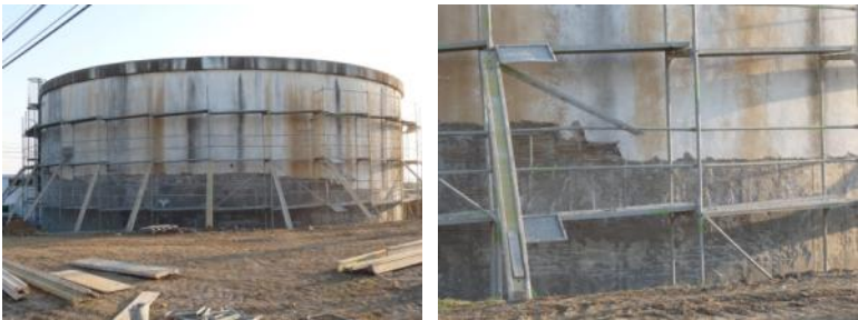
Removal of outside coating and storage tank waterproofing (after repair works)
