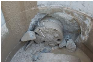
Exit shaft, head arrival
