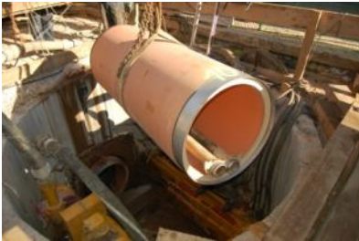
Pipe section installation
