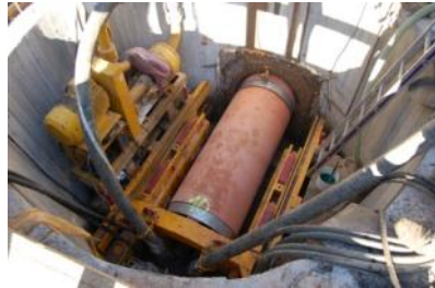
Initiation of pipe pushing
