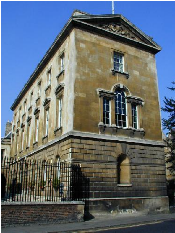
Imagen 173: First Court, Buroughs Building
