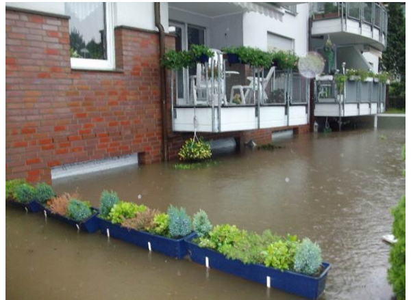
Figure 3 Urban Flooding after extreme rainfall event, Bochum Harpen
