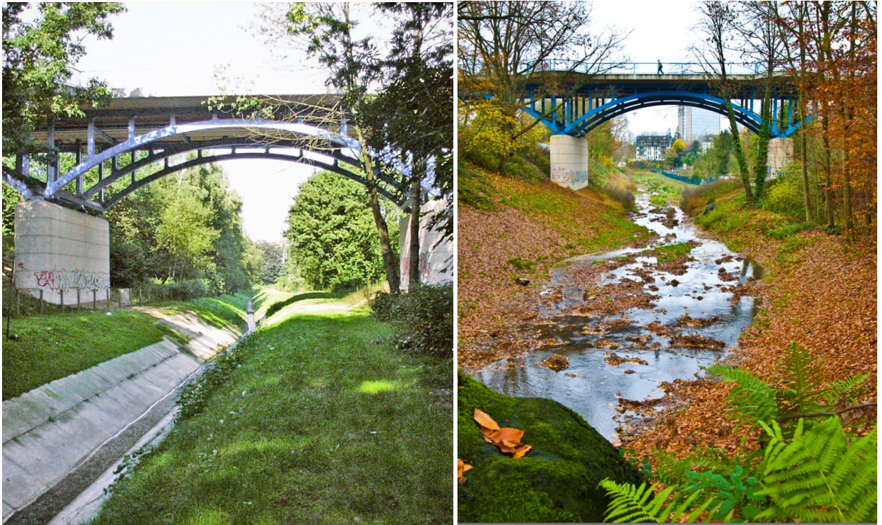
Figure 1: The Borbecker Mühlenbach as a concrete open wastewater sewer (left) and one year after the ecological improvement (right)
