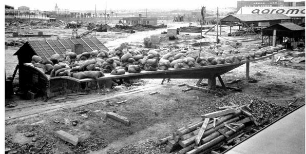
FIG. 2.34. MODELO A ESCALA REAL DE UNA LÁMINA
