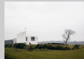
Fig 197. Vista exterior general
