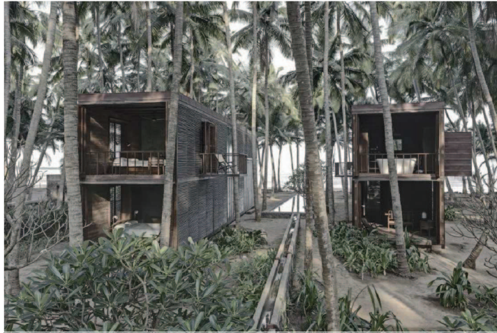
PALMYRA HOUSE. STUDIO MUMBAI. 2007. NANDGAON, MAHARASHTRA.
