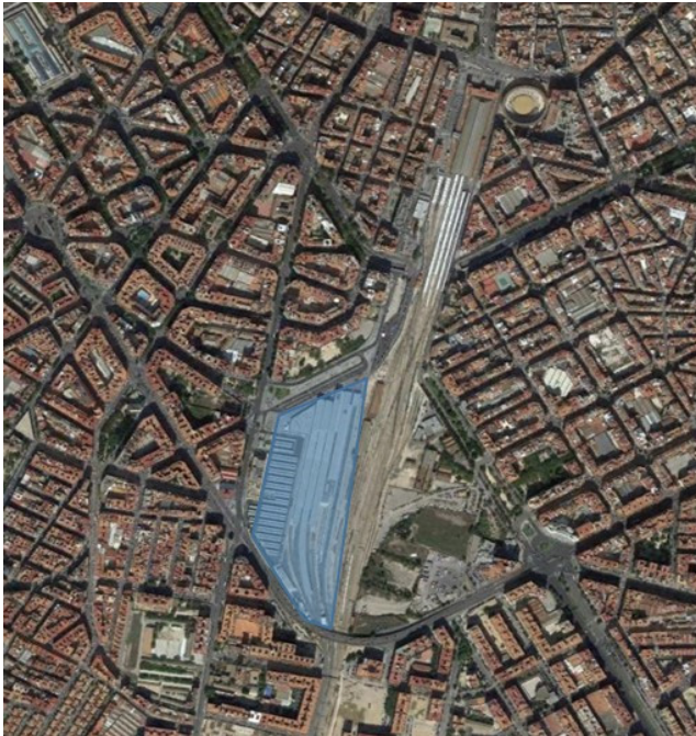
Figure 10: High-speed rail of Valencia, temporary station from 2010. (Source: Google and author.)
