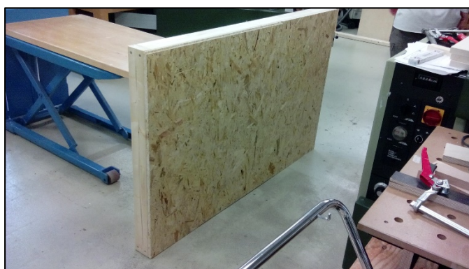
Picture N° 8: Panels construction. (The Author, 2015)
