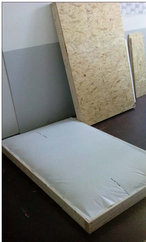
Picture N° 6: Insulating material added to the timber frame. ( The Author, 2015 )
